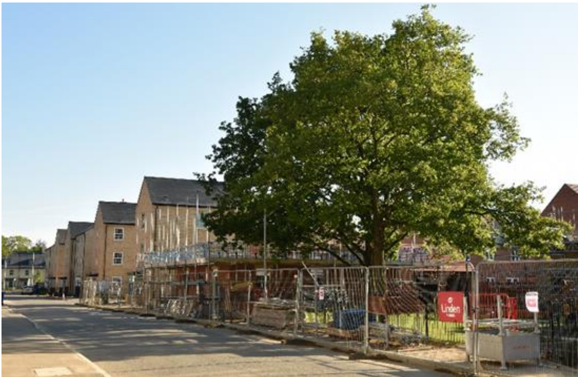
Forster Road, Brampton (HDC)
